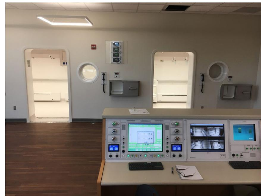
**Figure 2. Photograph of the inside of a rectangular multiplace hyperbaric chamber showing the fire deluge system, communications apparatus, internal surveillance, entertainment, medical lock, gas supply ports, view port, environmental control systems.** Supplied by Fink Engineering.
