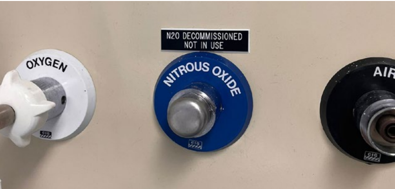
ABOVE FROM LEFT Decommissioned N 2 O wall outlet. Portable nitrous trolley system for PRN connection.
